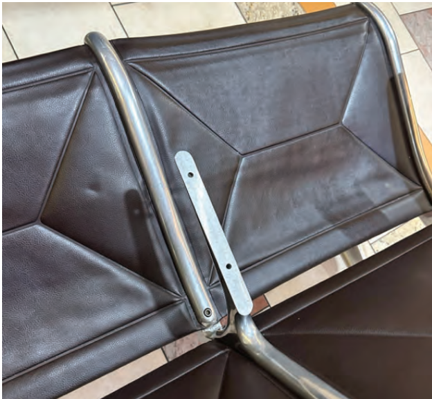
Seat missing arm rest located outside of T2 level 3 checkpoint B. Information desk agent on the east end has the armrest to reattach.
